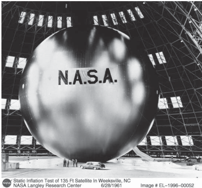
Figure 6.3 NASA Echo-I balloon project tested on the ground. Credits: NASA.
